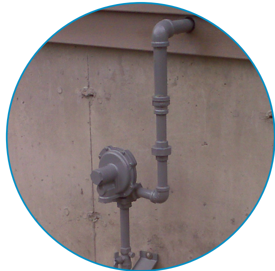
Example of a secondary pressure regulator
